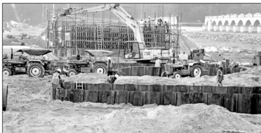
Figure 7: Sheet pile - combined pile system
