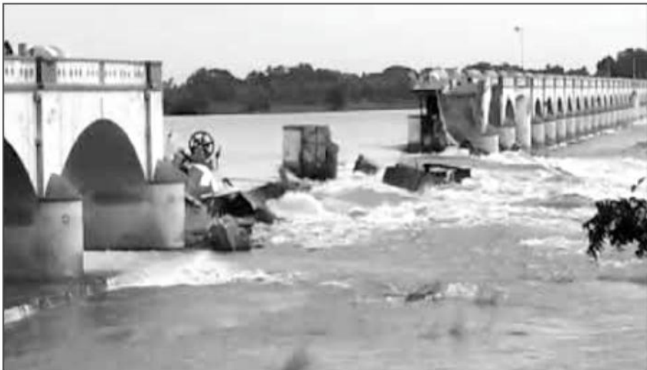
Figure 2: Collapsed Regulator
