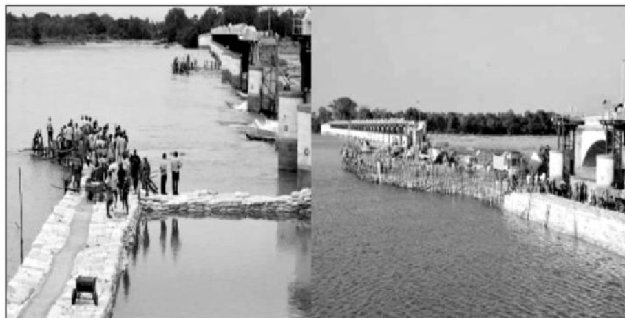
Figure 6: Cofferdam Construction
