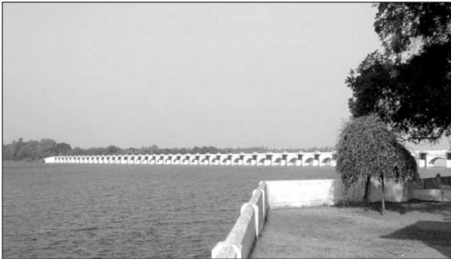
Figure 1: Upper Regulator Before the collapse
