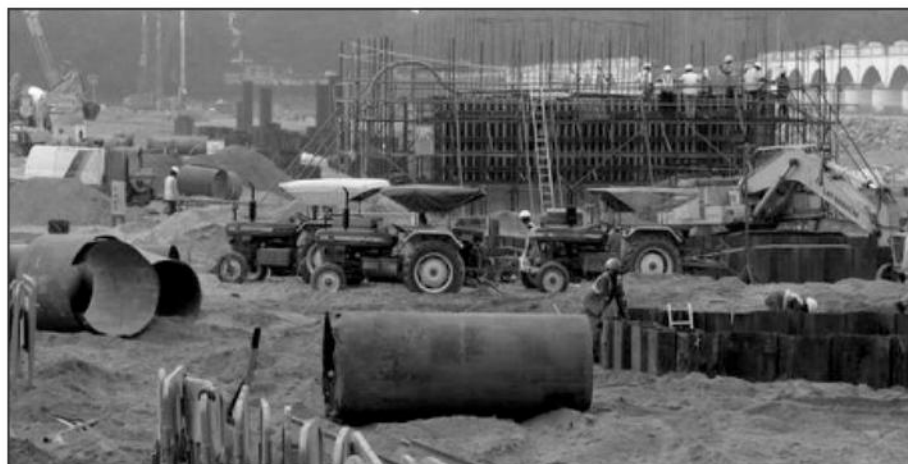
Figure 8: New Regulator construction
